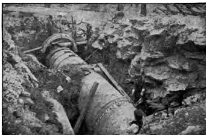
FIG. 16.—REPAIRING 6-FT. MAINS.
